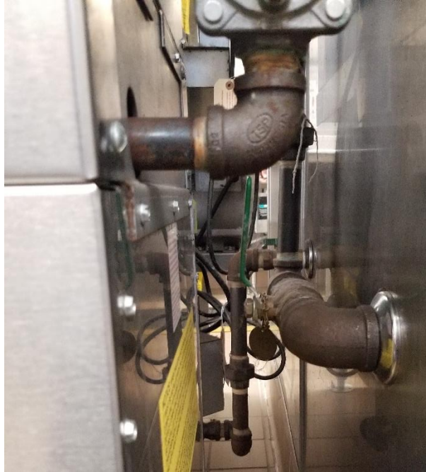
Figure 6. Gas appliance connections in the kitchen.
