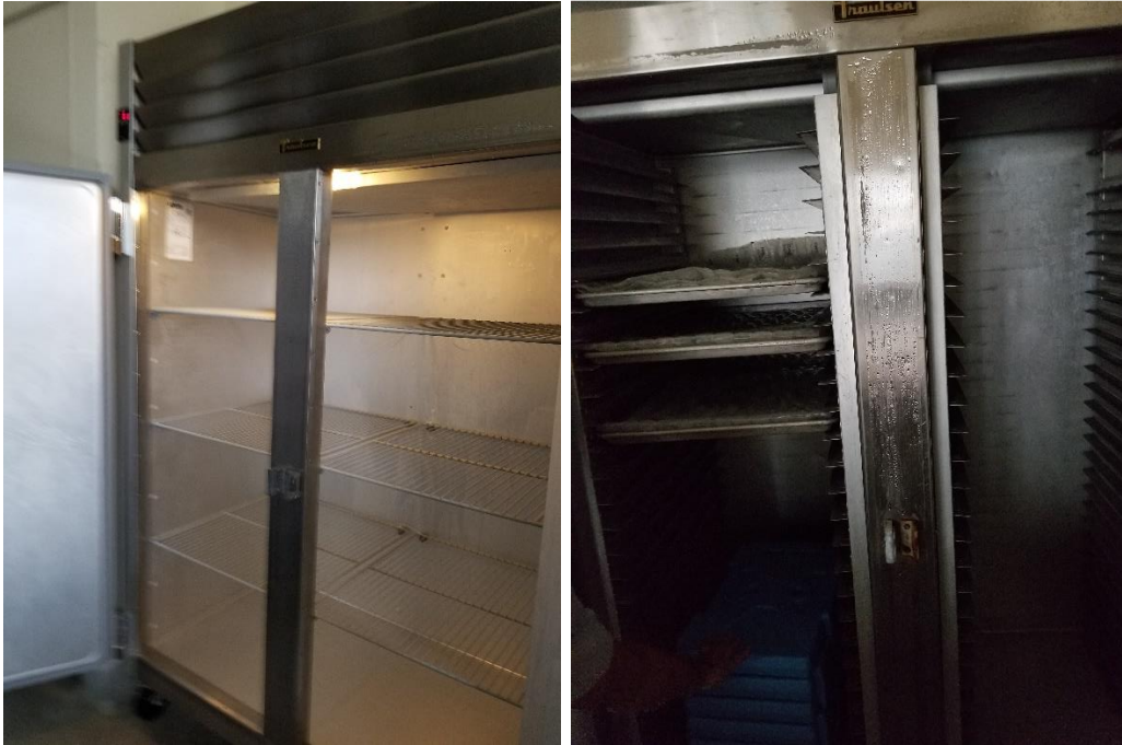
Figure 7. Commercial Refrigerator and Freezer left plugged in while empty and not being used. It is recommended to have these unplugged, emptied, and cleaned out while occupancy at the school is limited and common areas are not being used.
