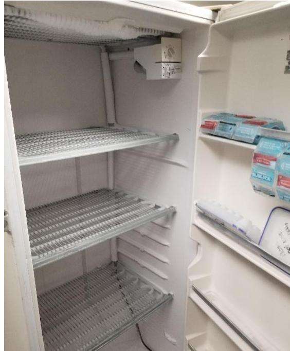
Figure 9. Older freezer left on and plugged in. It is recommended to have these unplugged, emptied, and cleaned out while occupancy at the school is limited and common areas are not being used.
